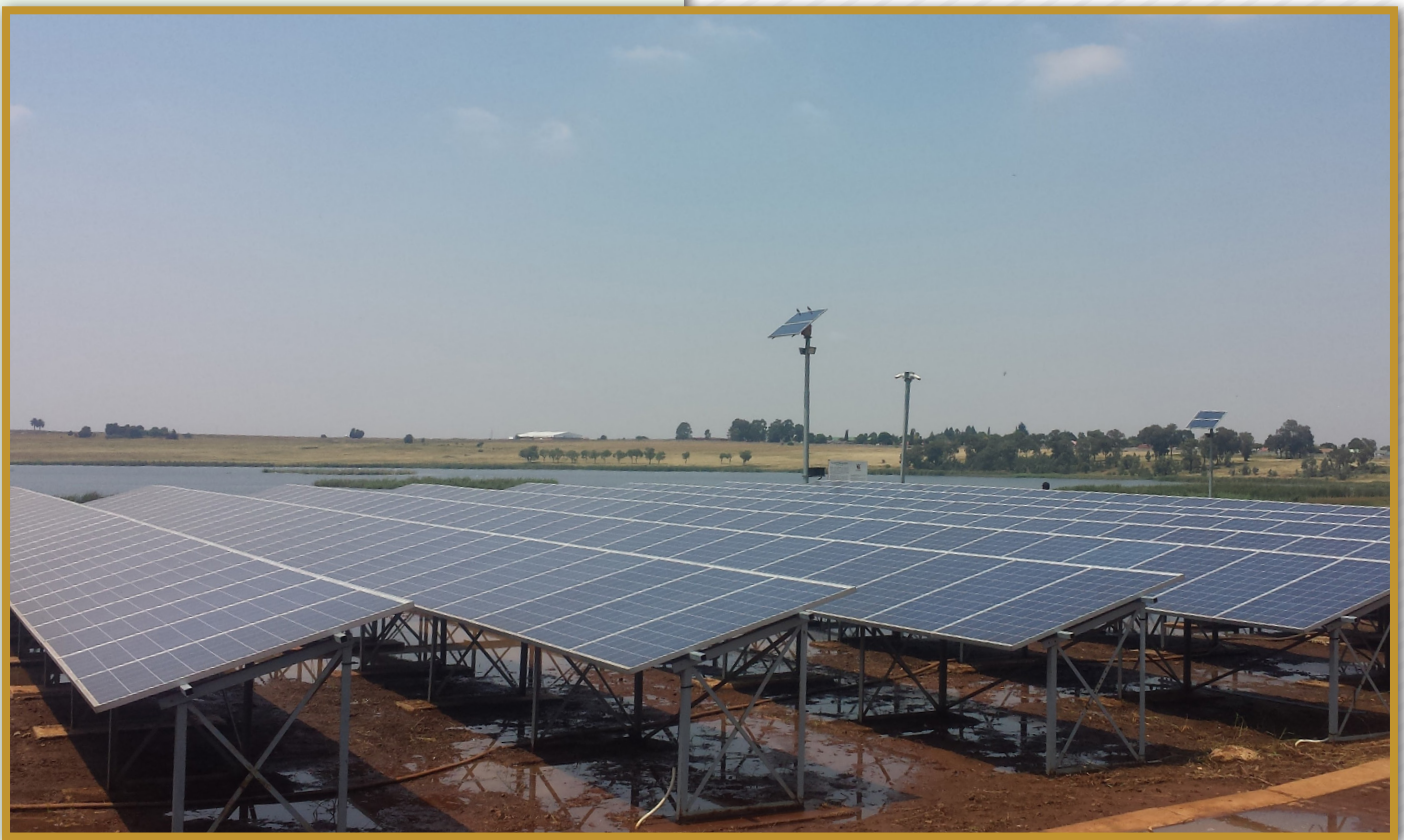
The solar panels Source: Energy Department: Alternative and renewable Energy, Ekurhuleni Municipality
