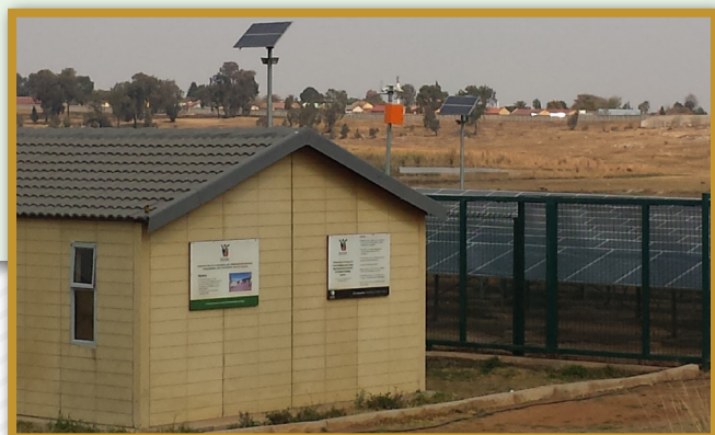
The power house containing the inverters (amongst others) Source: Energy Department: Alternative and renewable Energy, Ekurhuleni Municipality
