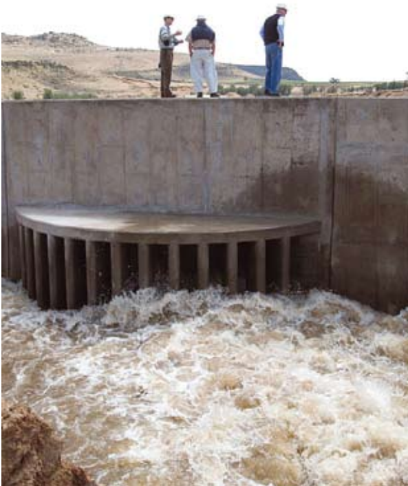
Fig. 1: Merino intake works.
